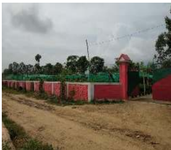
Ngangkha Nursery Fencing, Bishnupur under CAMPA
